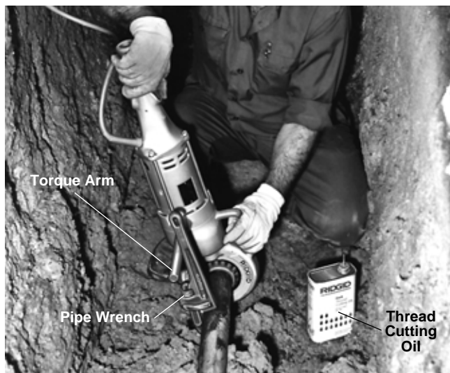
Figure 6 – Ideal for Construction Use
